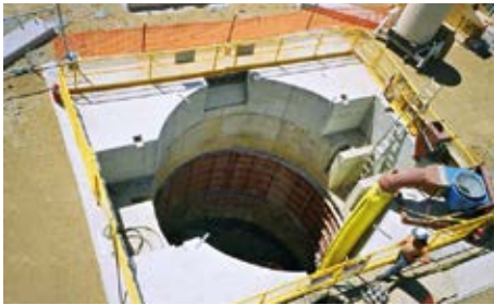
Shaft collar for a 6.3m diameter raise bored shaft.
