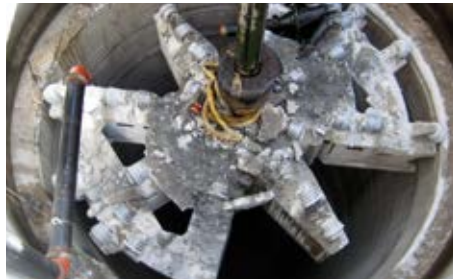
Breakthrough of a 6.3m diameter reamer into the shaft collar.
