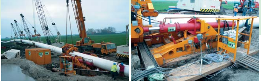
Pipe Thruster installed at the launch pit.
