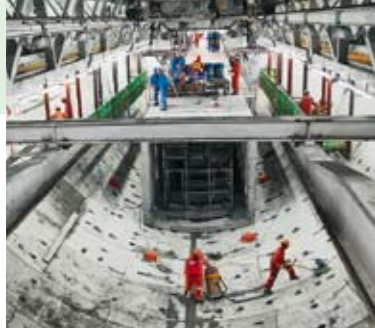
Tunnelling work of the S-317.
