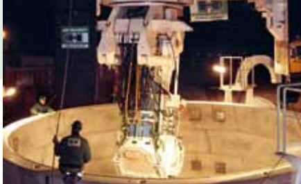
Installing the VSM9000 at the construction site.
