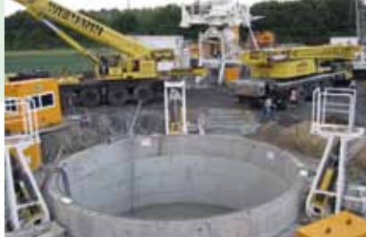
23-meter deep shaft was sunk in 17 working days.
