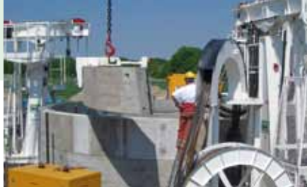
Shaft sinking and shaft lining carried out simultaneously.
