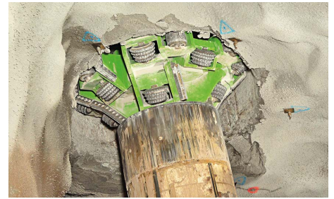
Breakthrough of reaming head.
