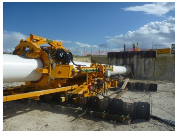
The Pipe Thruster provides up to 500 tonnes of thrust force at the launch side.
