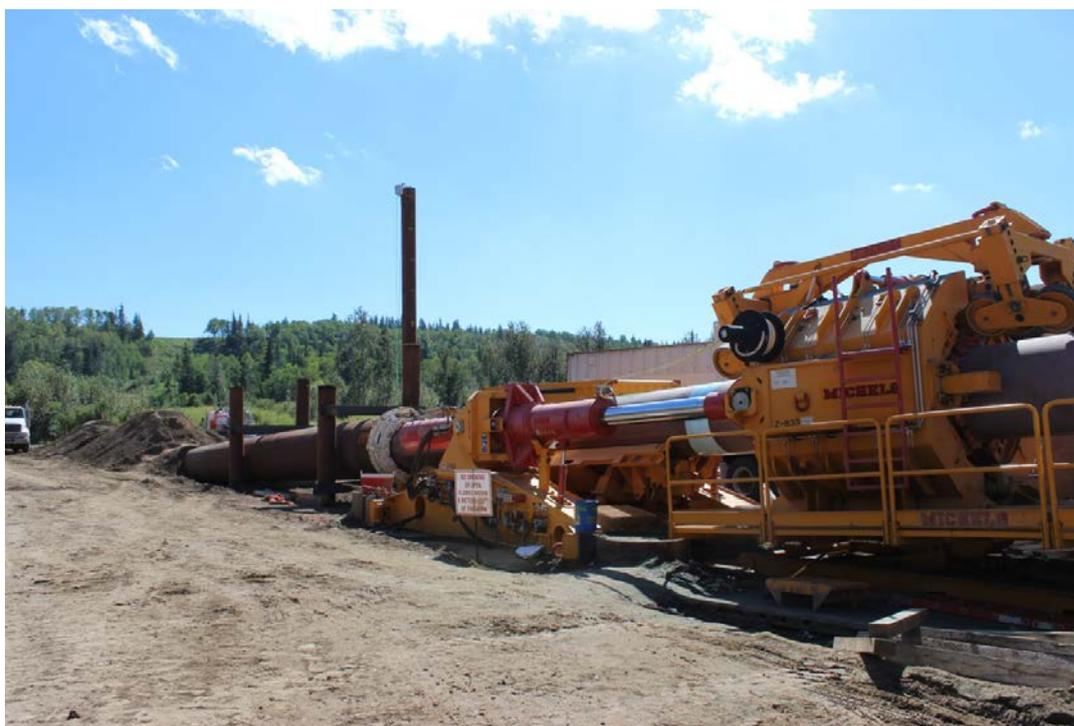
Pic2\_ Direct Pipe® Technology from Herrenknecht allows for the installation of a prefabricated pipeline in the trenchless mode in only one work step, while the required borehole is excavated simultaneously. This provides for the speedy and highly cost-efficient installation of pipelines with lengths of up to more than 1,500 meters.
