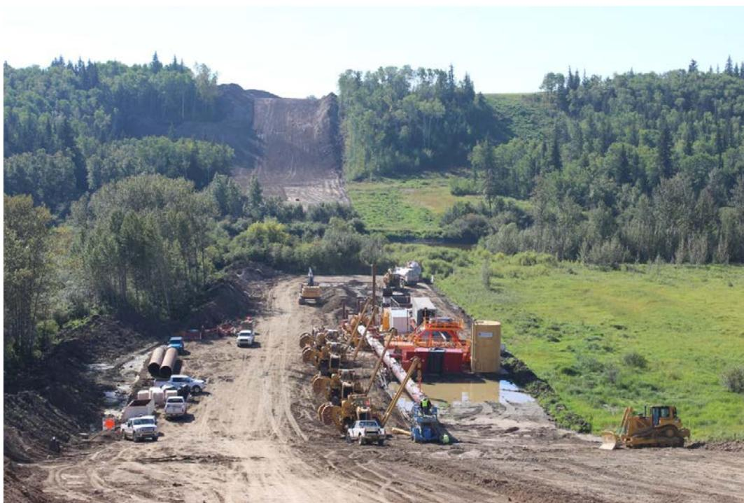
Pic1\_ Direct Pipe® technology premieres in Canada: A pipeline with a diameter of 42 inches (1,067mm, double FBE coating) was built over a length of 340 meters under the Beaver River in the province of Alberta in only 13 days.
