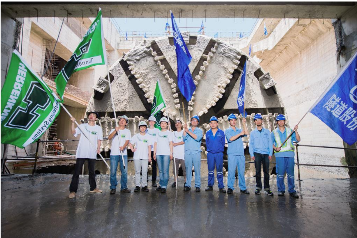
Picture 3: Final breakthrough on June 19 th , 2013: S-569 (Ø 15 430 mm) successfully completed West Changjiang Road River Tunnel.
