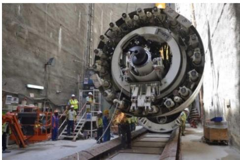
Site assembly of the Herrenknecht tunnel boring machine which is the first TBM to drive a tunnel in a segmental lining process in Qatar. Apart from the two machines for the Abu Hamour Southern Outfall waste water project, the Emirate will also be deploying another 21 Herrenknecht EPB Shields during construction of the Doha Metro.
