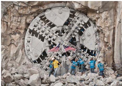
Breakthrough of the first Variable Density machine on January 9, 2014: the TBM developed especially for the Klang Valley MRT project combines the advantages of EPB shields and Mixshields. The ability to adjust the suspension density in slurry mode expands the potential application range and makes the machine an all-round solution for loose rock advances of all kinds.
