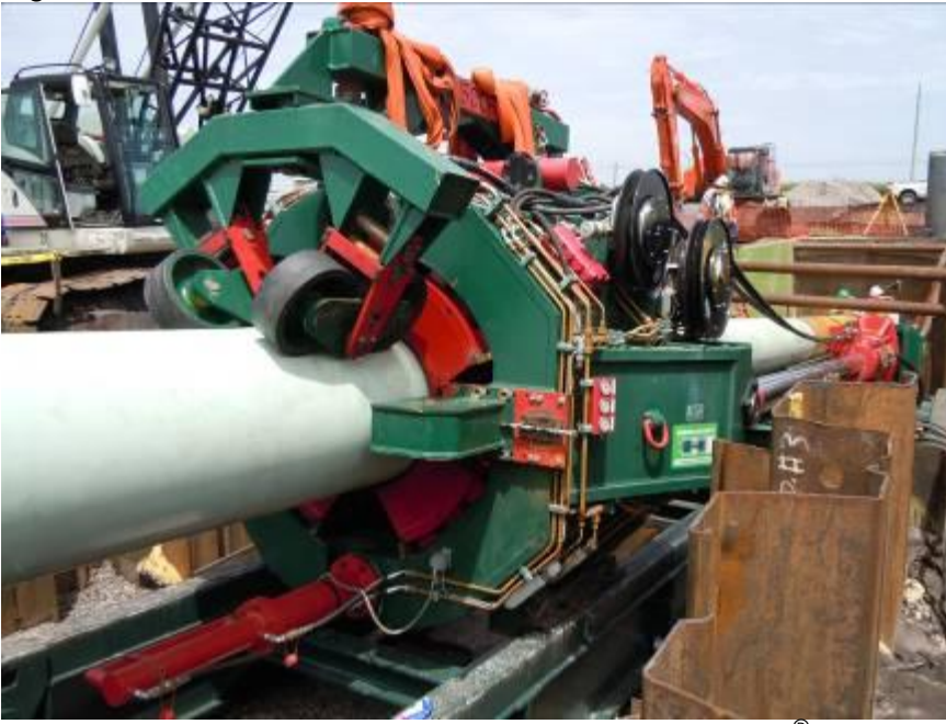
The Herrenknecht Pipe Thruster pushes the Direct Pipe ® machine and pipeline forward with an average thrust of 15 tonnes.
