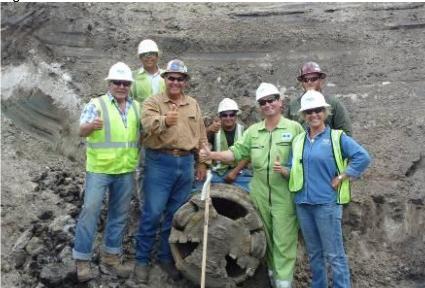
Breakthrough on August 29, 2010 after only three days (single shift operation).
